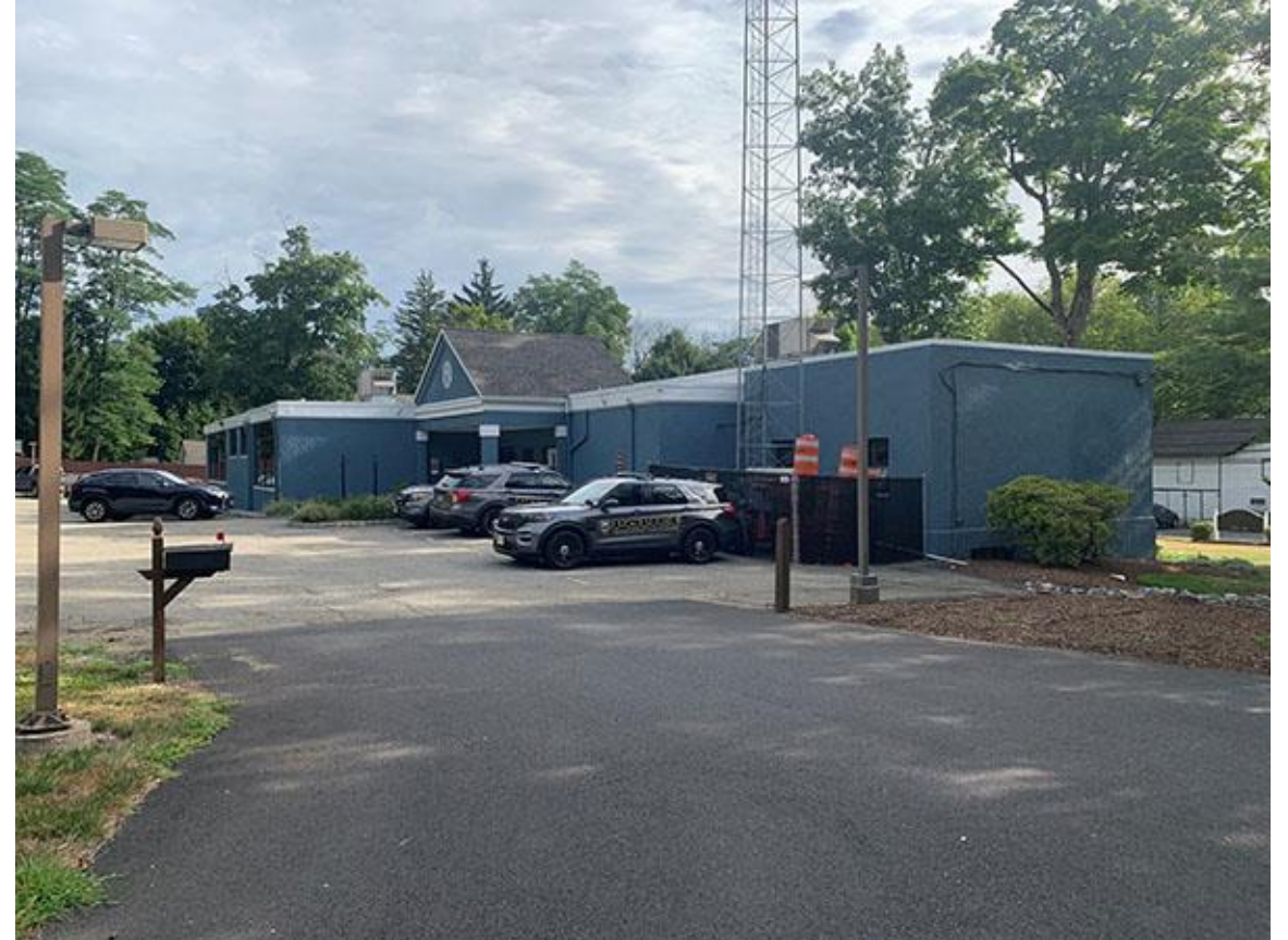
1972 + 1997 Additions: Main Building Entrance, No Sallyport, Lack of Storage for Road Items
