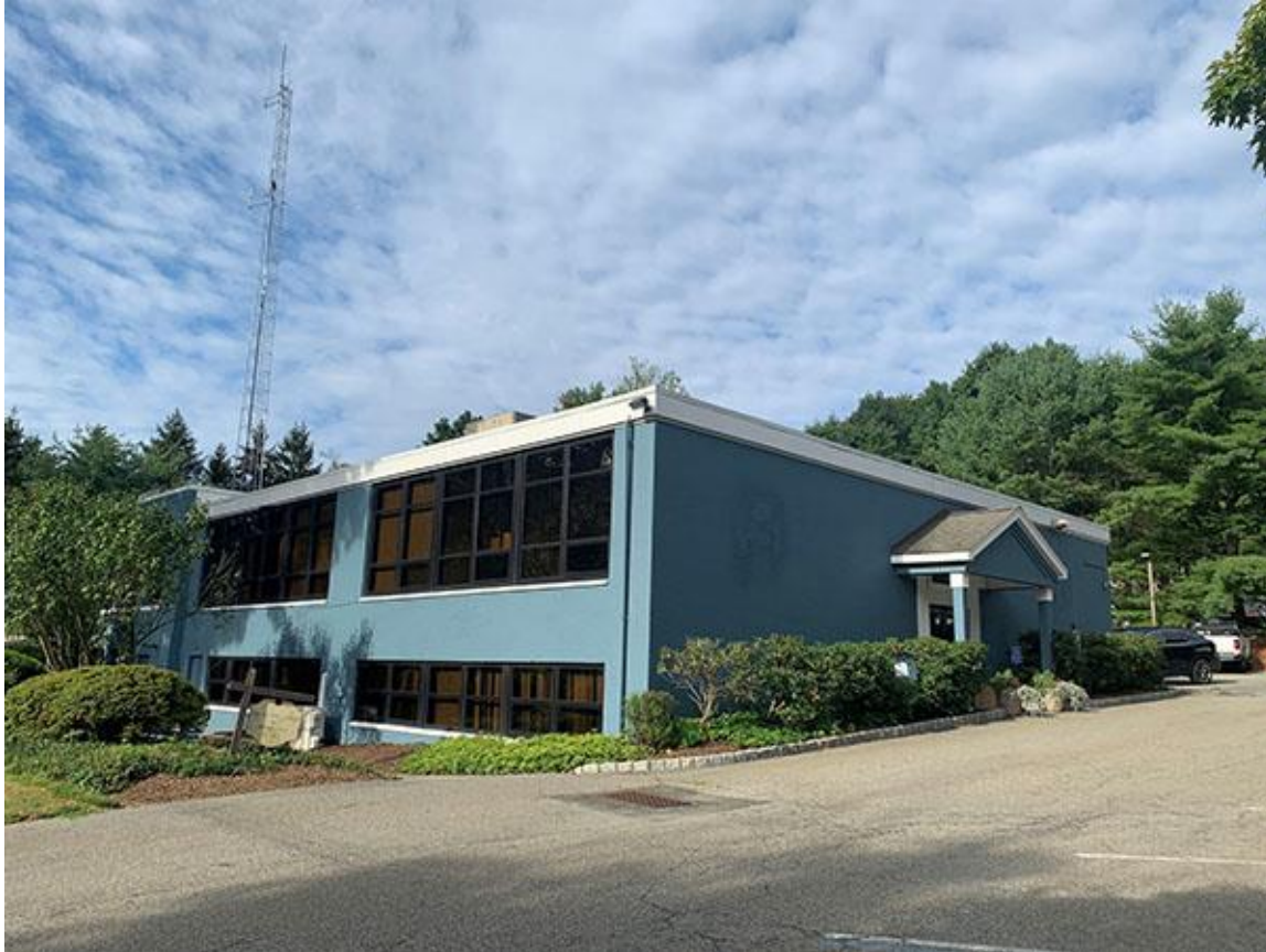
1952 Addition: Glass at Dais Area, Communications Tower
